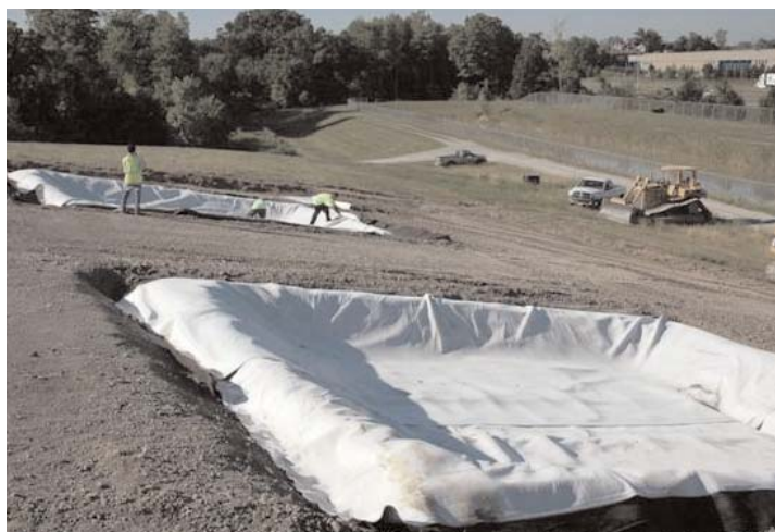
Field-Scale lysimeters constructed at Woodland Meadows Landfill, Detroit, Michigan
