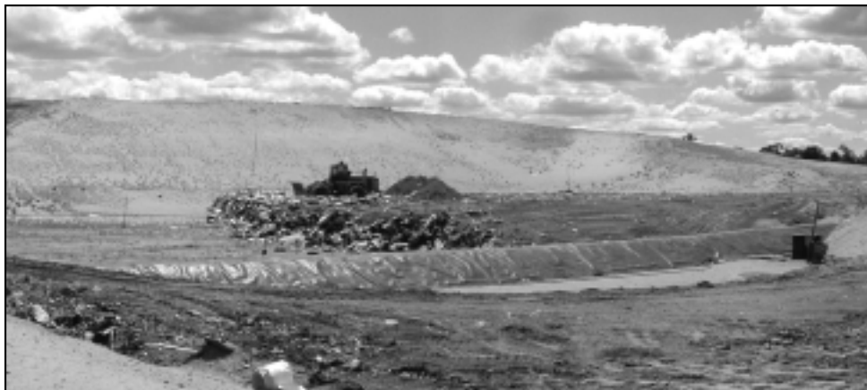
EREF's bioreactor project received its first lift of waste in August 2002.
