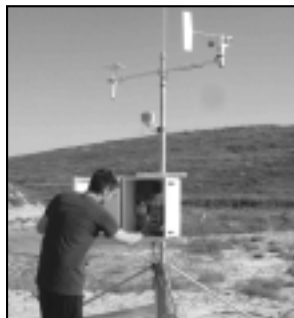
Weather monitoring station is installed on the perimeter of the bioreactor cell.
