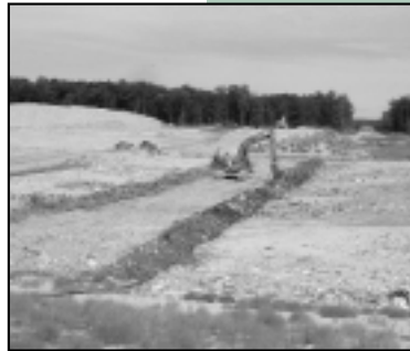
Settlement profilers are lowered within the first lift of waste.
