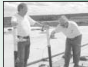
EREF Vice Chairman Bob Stearns (right) examines a gas monitoring riser on the landfill. Ed Repa, EREF, is more than happy to let Bob take the lead.
