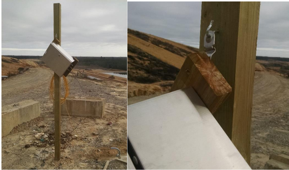
Figure 4-29. Flexible Mounting and Extra Cable for FODTS Readout Box to prevent damage from settlement of waste.
